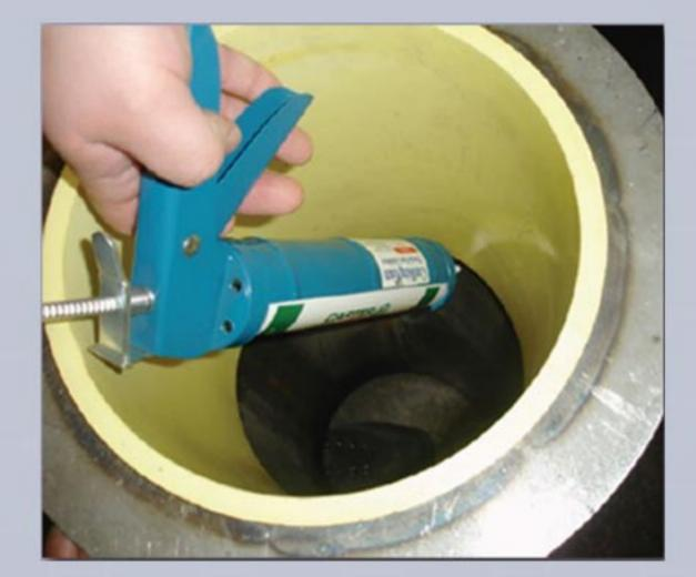
Then, simply add a bead of silicon caulking to the bottom of the transition sleeve to limit water and debris from collecting behind the sleeve.
