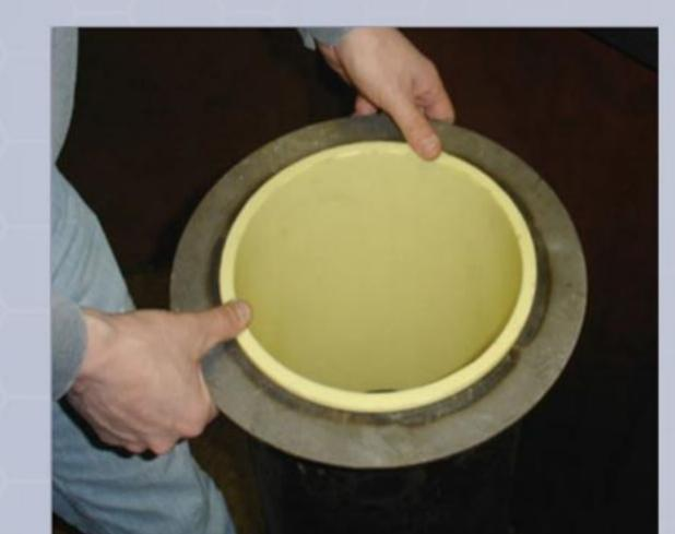
Simply slide the sleeve into the existing steel transition tube so that the ring on top sits on top; as seen here.
